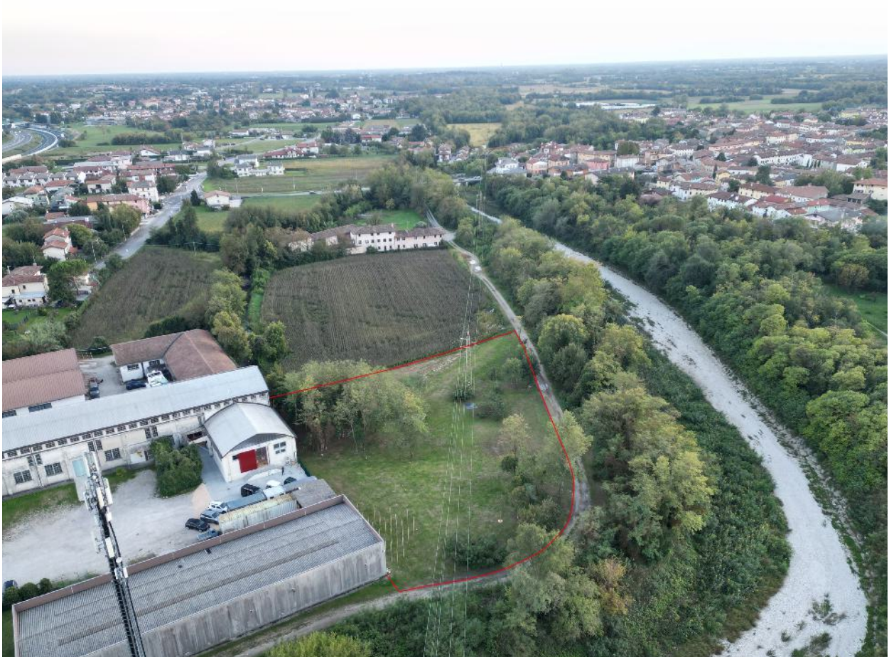
Aerial view of the site
